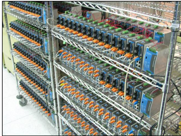
Figure 15: Recovery time testing with a large number of switches
